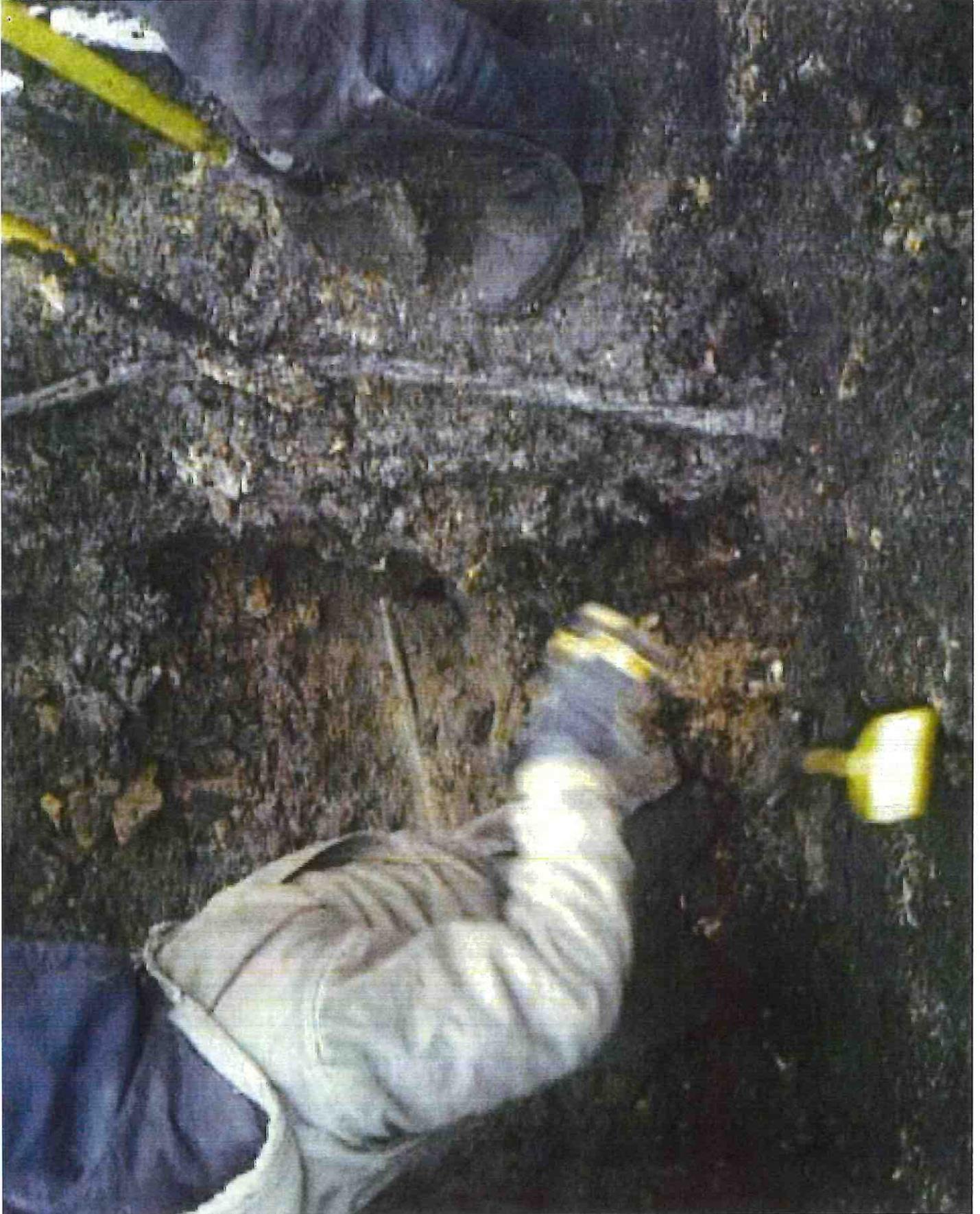
PLASTIC USED TO POUR CONCRETE ON P.E./CLAY JOINT
